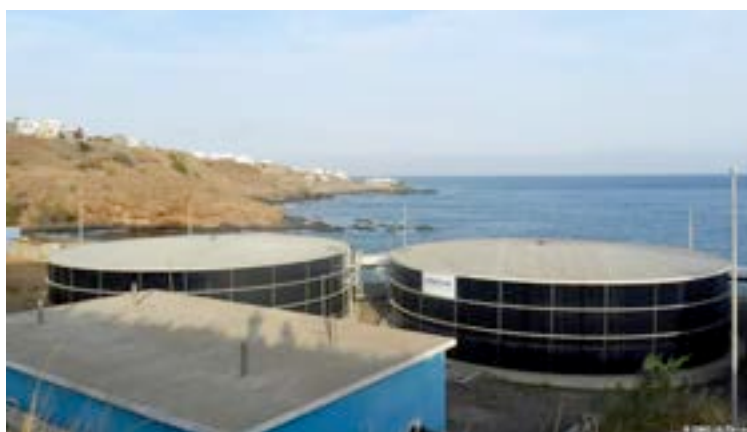
Desalination station in Cape Verde. Source: DW / V. Teixeira.
